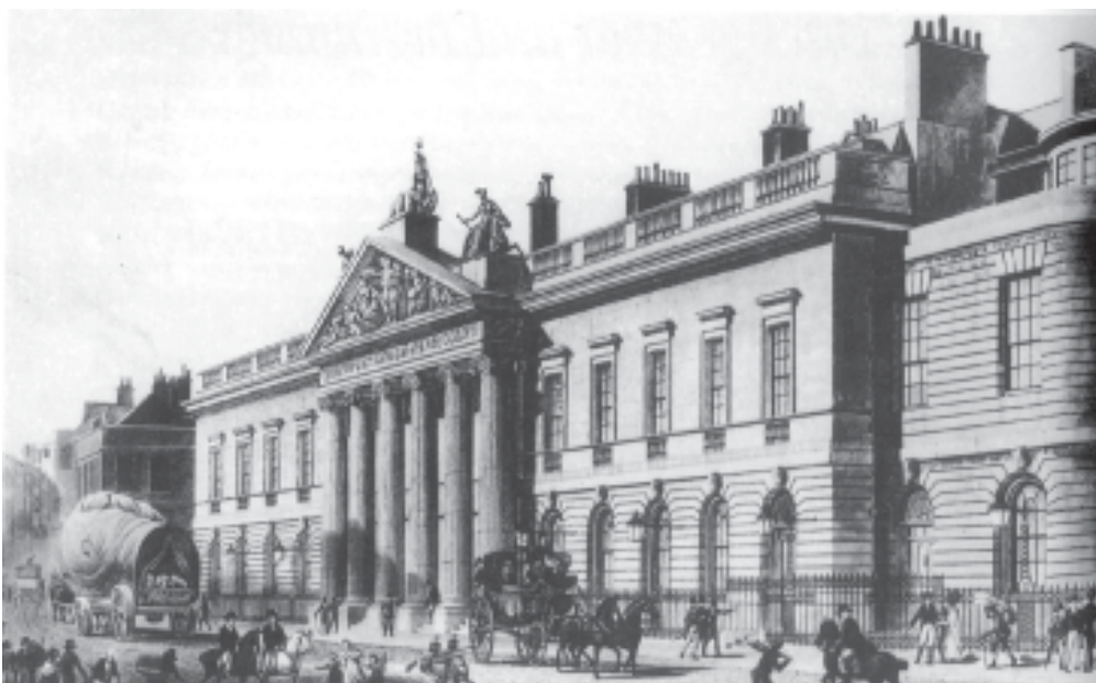
Fig. 17 – East India Company House, London.
